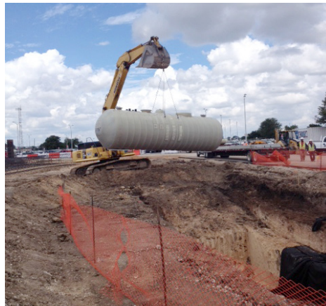
Austin Commercial places the 10,000 gallon oil water separator in the service yard. The oil-water separator is located along the eastern wall of the service yard and is intended to catch and separate any sedimentation or hazardous type of materials upstream of the main City of Austin storm sewer system.
