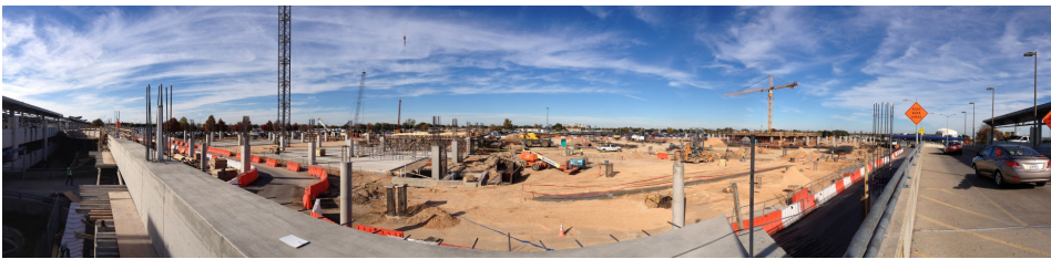
Tower Cranes and foundation work can be seen in this panoramic view of the project site from November, 2013.
