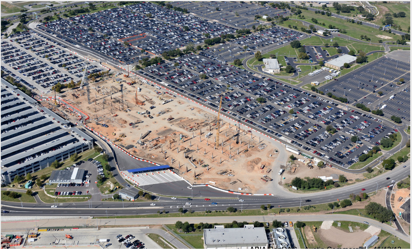
This aerial view shows the vertical construction that has begun on the Consolidated Rental Car Facility. Tower cranes have erected dozens of standing columns which will support the building structure.
