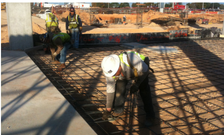
Workers lay foundation reinforcement for the main footprint of the Consolidated Rental Car Facility.
